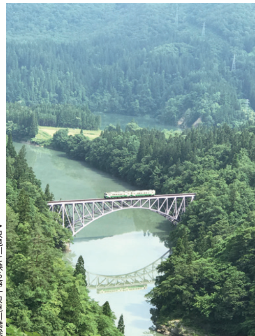
▶只見川に映る第一只見川橋梁
