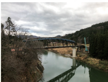
▶第七只見川橋梁の復旧工事
